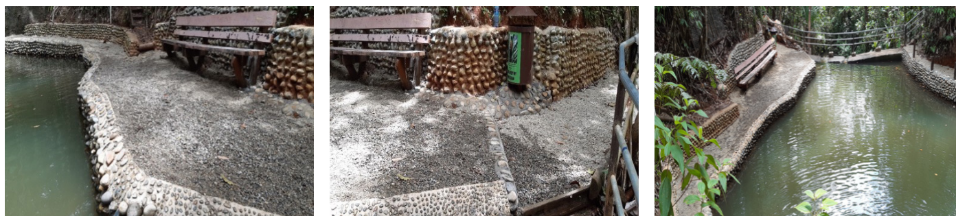
Figure 6: Rock lining on both sides of the 1st pool and also on the walkway and side walls.
